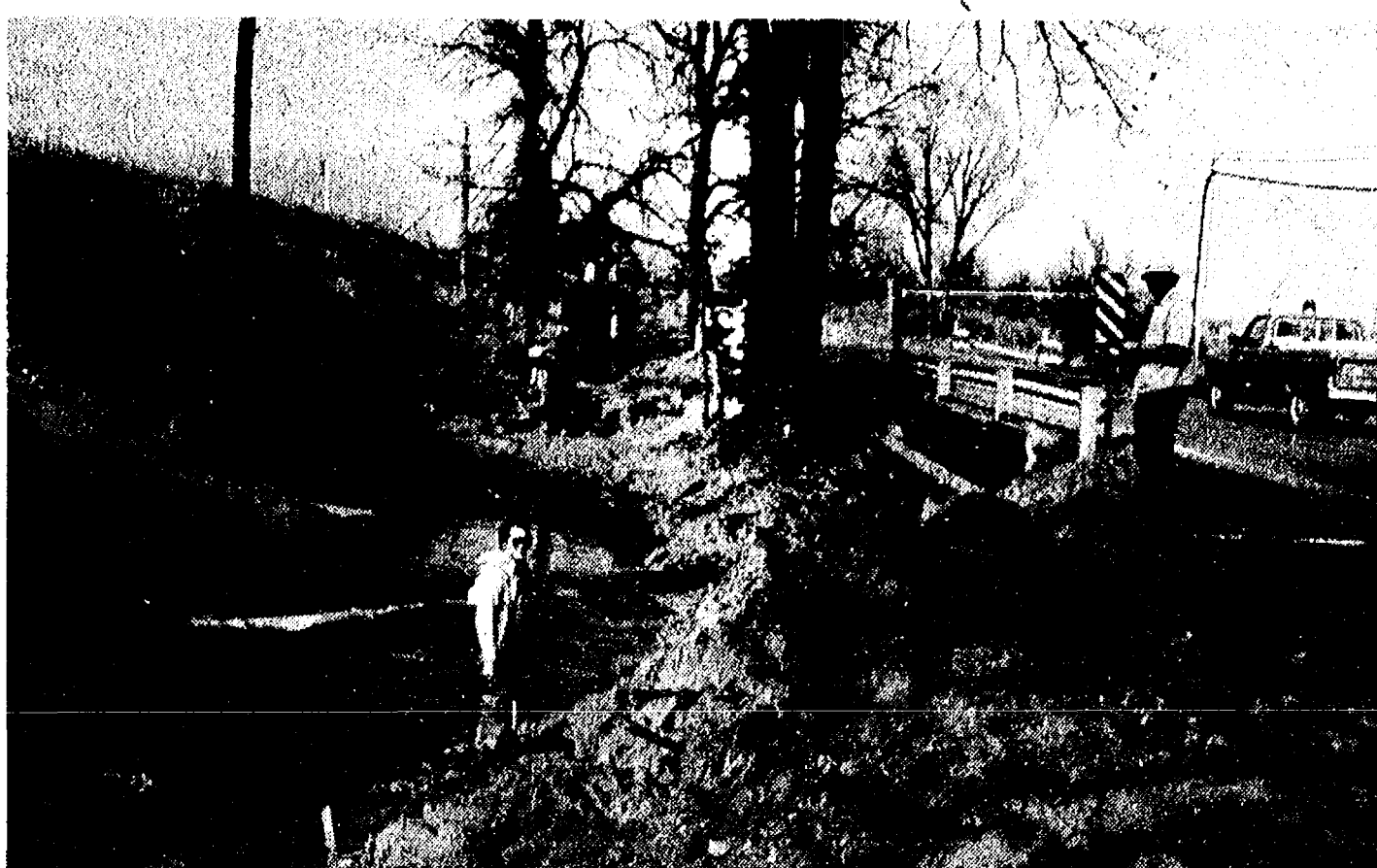
BRIDGE WORK BEGINS—Chelsea-Dexter Rd. between Freer and Lima Center Rds. was closed to through traffic beginning yesterday as work started on replacing the bridge over the north fork of Mill Creek.
